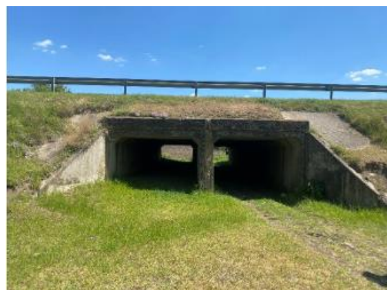
Fig. 7-2: The general view of the bridge Lot no.2
