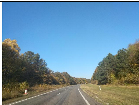
Fig. 7-4: Bursuc area, approximately km 44
